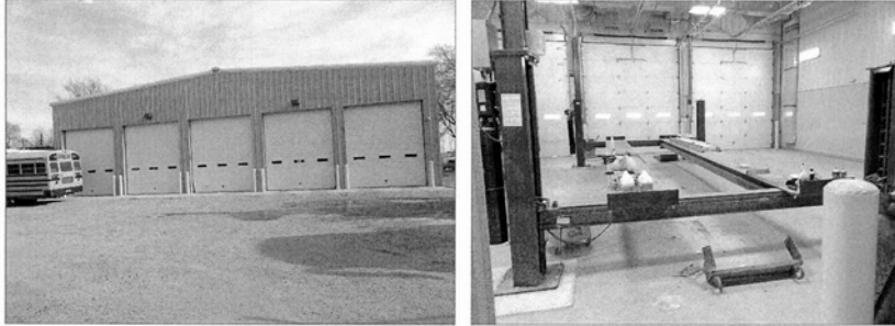
Figure 6: Exterior and Interior of Recently-Constructed Bus Maintenance Building Where Door Does Not Close When a Large School Bus is on Hydraulic Lift
