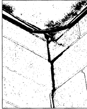
There are many severe cracks inside the academic buildings, which could cause wiring to short-circuit.
