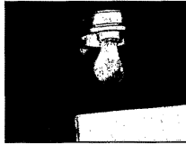
Exposed light fixture in locker room shower can electrocute the students.
