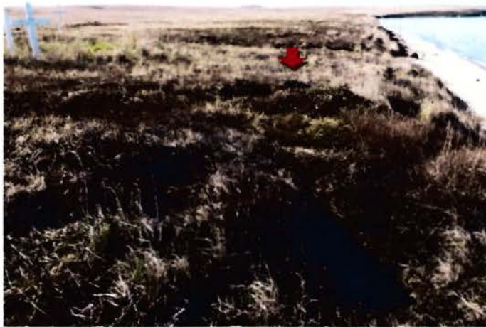
Looking southwest away from Teller. Cemetery edge on left. Looking straight into the “slump zone” that is full of cracks in the ground, and is slanting down towards the beach.
