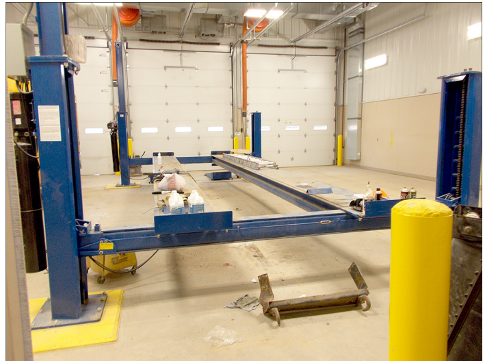
Figure 6: Exterior and Interior of Recently-Constructed Bus Maintenance Building Where Door Does Not Close When a Large School Bus Is on Hydraulic Lift
