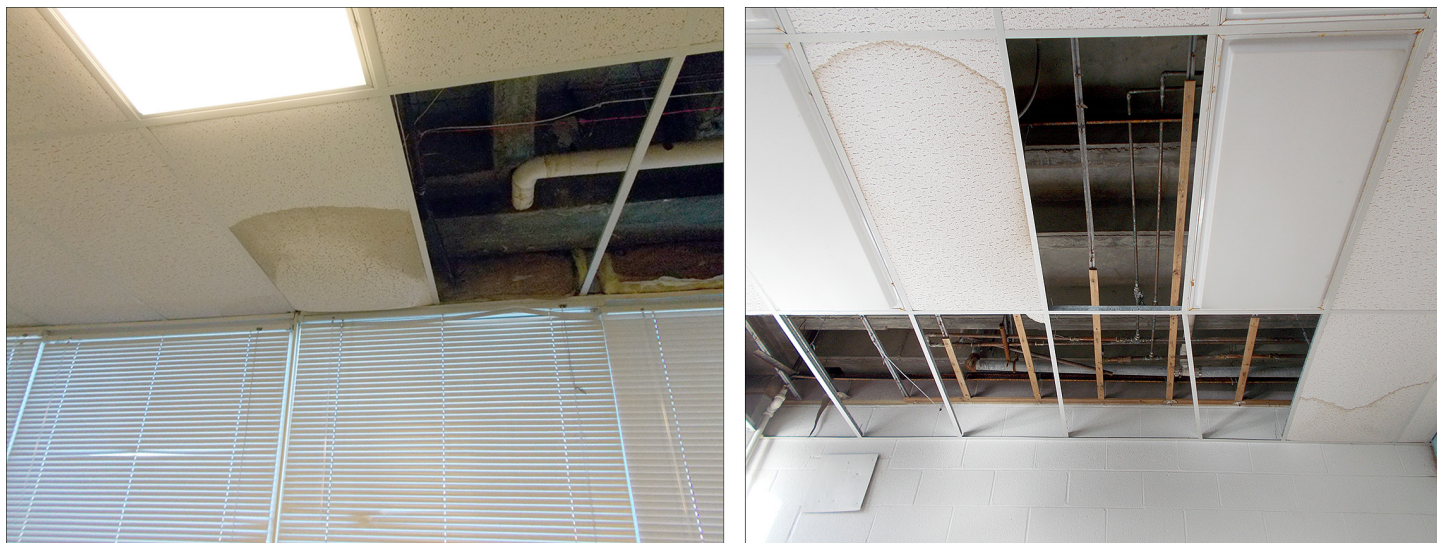
Figure 5: Damaged or Removed Classroom Ceiling Tiles Due to Leaks in Recently-Installed Roofs
