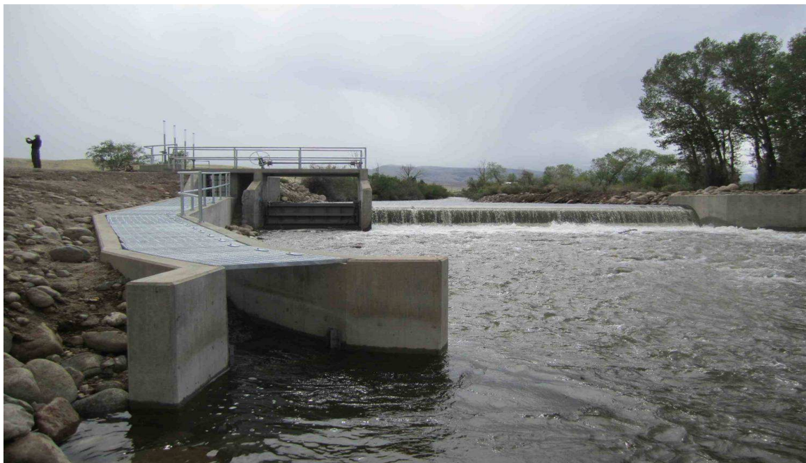
Ray Canal Diversion Structure and Fish Passage
